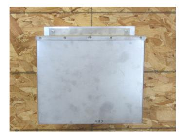
Center the outside cover on the stainless steel thimble face, mark the holes and drill pilot holes with a small drill bit. Secure the cover using the provided 10 X 1" screws. You may have to use longer screws depending on the material on the outside of the house. Make sure you get into solid materials with the screws so your fan and cover are well supported.
