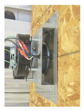
This is the view of the electrical cord coming out the house wall, through the grommet in the thimble face, through the grommet in the adapter plate and hooked up to the motor connections. Fish the wires through before putting the connectors on the end of the wires. You might want to put a small dab of silicone to secure the electrical wire to the rubber grommet to keep the wire from sliding out of the grommet.
